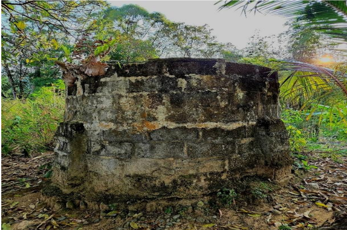
Figure 2. The first water reservoir
